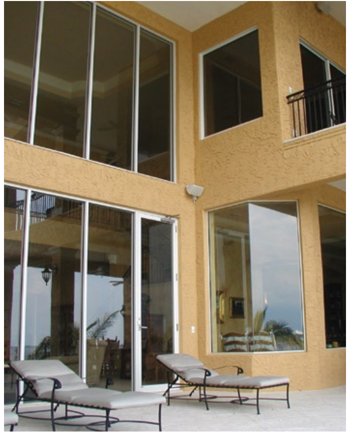
The immense windows of this home in Florida were retrofitted with Armorcoat solar safety film for protection from broken glass and hurricane season preparation.
